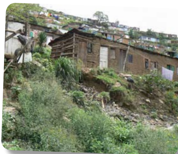
Informal settlement in Shayamoya, Claremont
