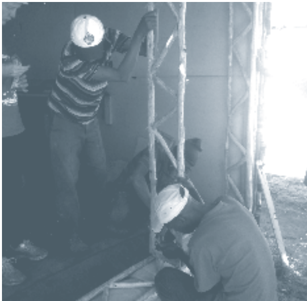
Setting up of a frame on the foundation – training day Zweledinga 17 September 2013
