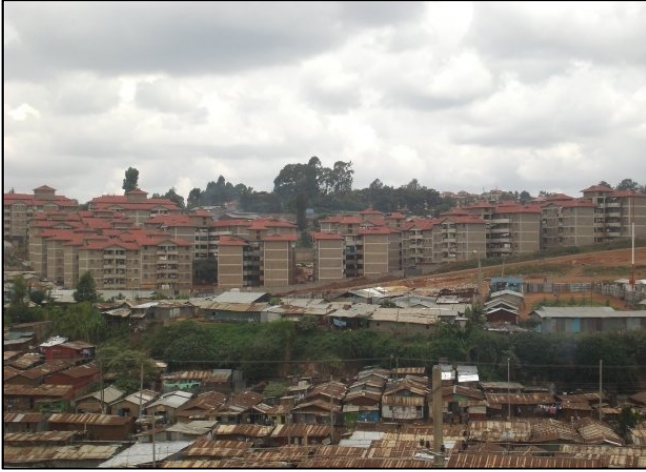
Fig. 7: Decanting facility in Kibera for residents who were living in the location where Phase 2 of KENSUP is being constructed, photo by Lene Le Roux, Sept 2012.
