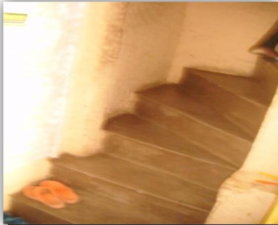
Fig. 15. Spiral staircase saving up space and construction materials.15/09/12. Photo taken by Pumla Bafo.
