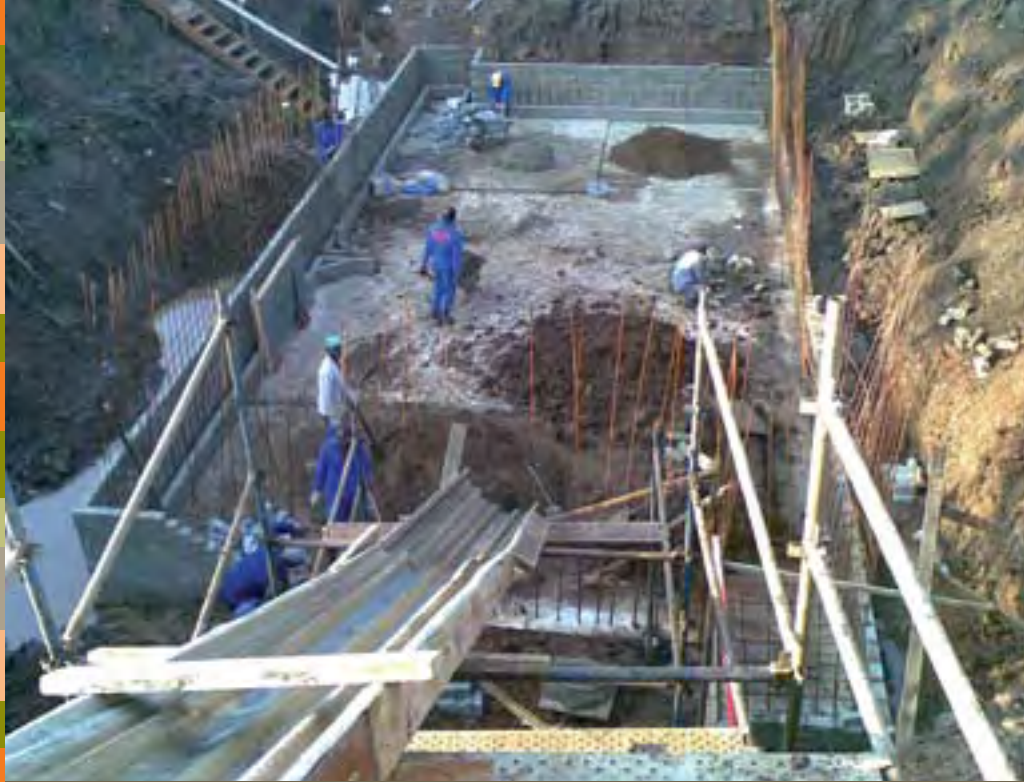
Clockwise from above left: Reinforcing of the digester in progress at Cato Manor, South Africa; The biogas power building and 1.416 MW Jenbacher gas gensets at Petro SA; Dry fermentation energy recovery plant in Moosdorf, Germany; Bran Sands Waste Water Treatment, UK.
