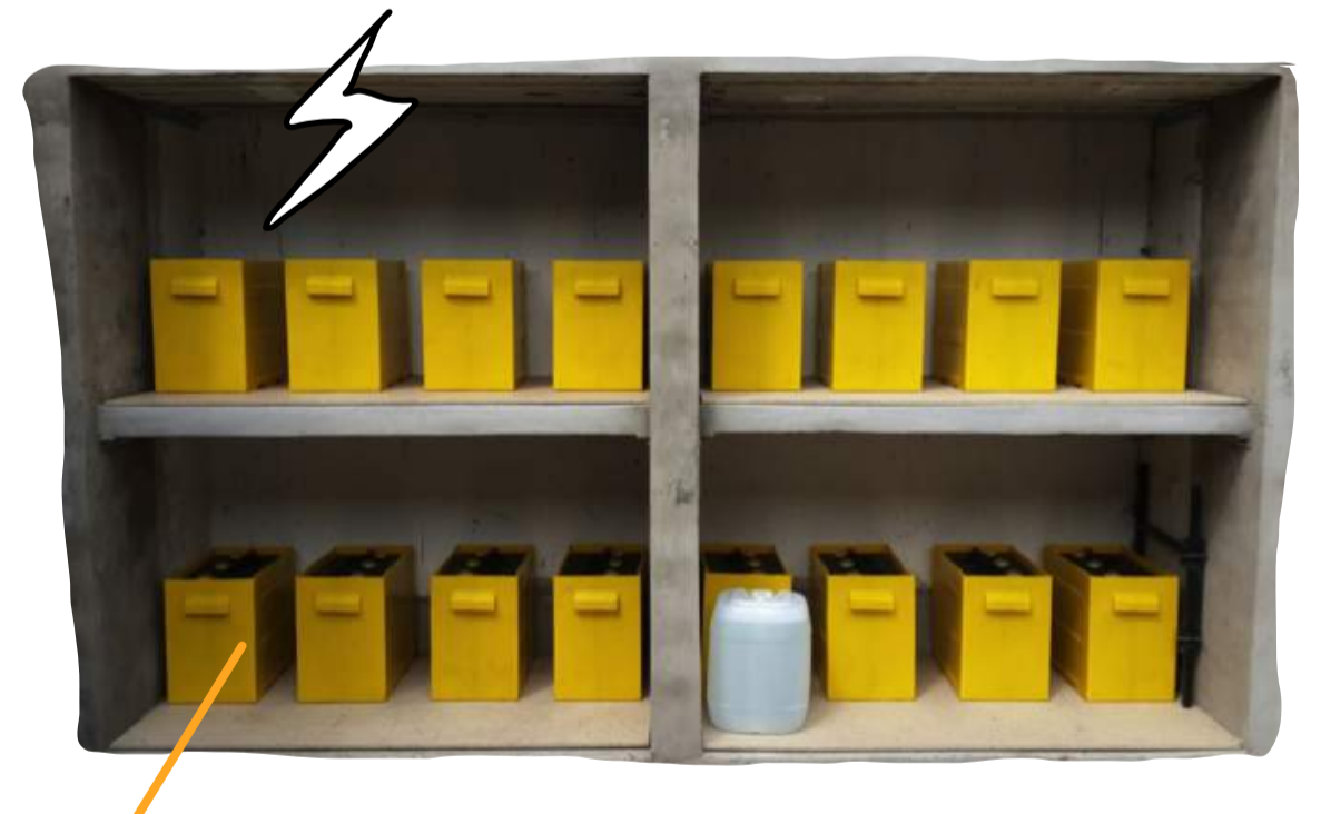
2 x 900ah battery bank for outages
