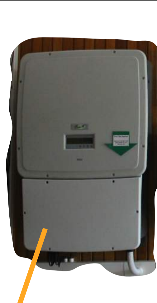
20kW Grid Tied ABB Inverter
