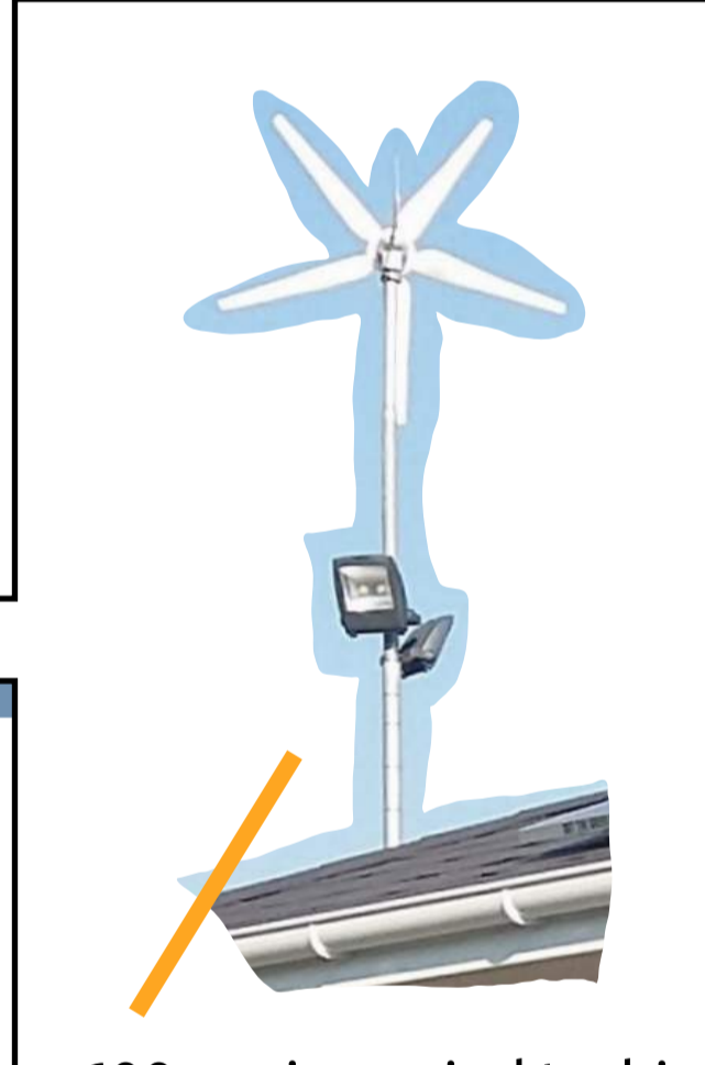
600w micro wind turbine will assist battery charging
